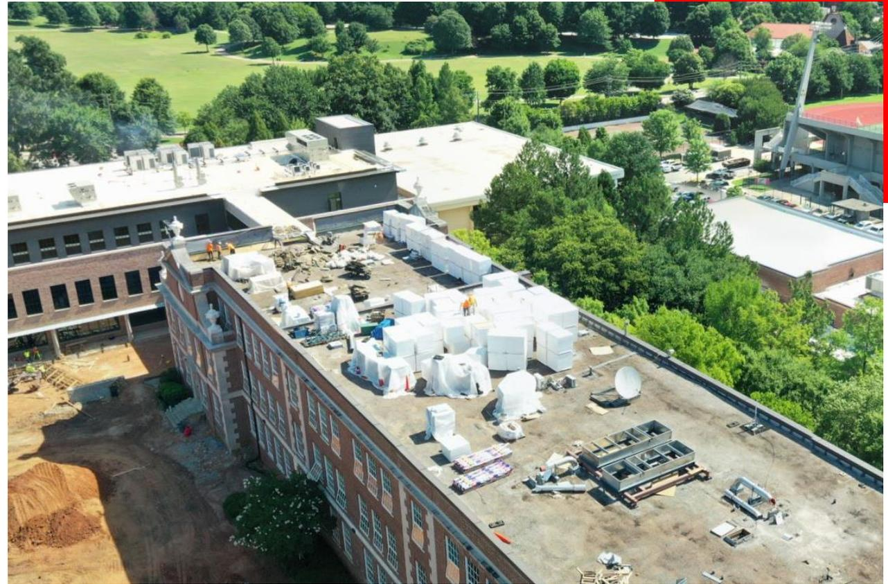
Charles Allen Building Rooftop Units Removed & Roofing Material Staged
